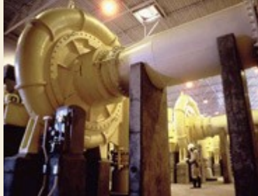
San Jose Water Pollution Control Plant
